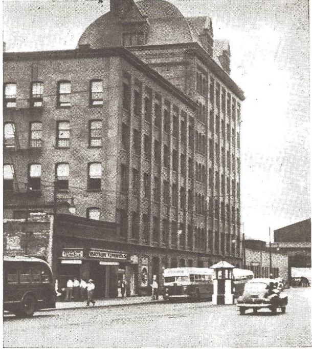
ONCE BUSY Exchange Place, PRR terminal, has few trains since Pennsy completed electrification of her mainline into New York City. Extreme right , ferry piers with entrance to H&M tunnels at far left
