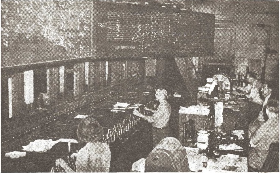
ABOVE: Scene in Pennsylvania Station (N. Y.) control tower shows illuminated diagram of track layout, with lights indicating train locations. Operators set switches by turning cranks. PRR pioneered in the installation of mechanical switch and signal interlocking plants
